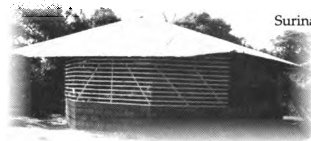
Construction of Gangasa village kitchen
