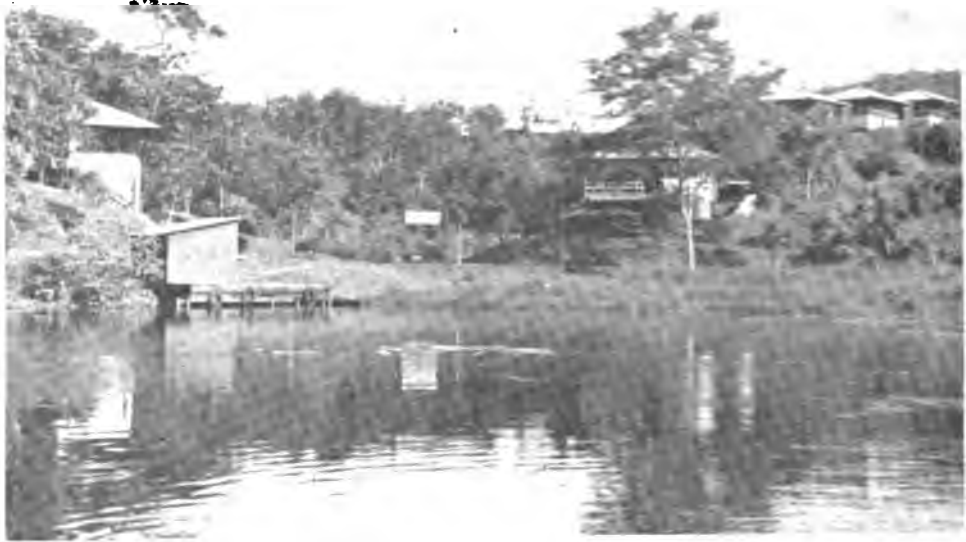
Dispensary, Store, and Three Laborers Cottages on Hill, Gasoline Shed and Dock at the Rubber Substation, Gatún Lake, Panama Canal Zone
