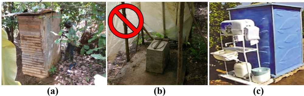
Photos 14 (a, b, c) Are these toilets adequate, appropriate, clean and well-served?
