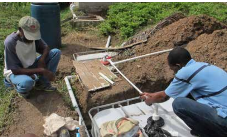
Establishing biodigester using water tanks at the demonstration plot.
