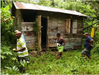
Assessments included Site Visits to map out local resources, inputs and skillsets available for enterprise development
