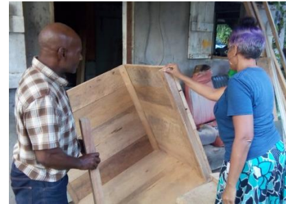
Building a Fermentation box: opportunity was taken to build relationship with skilled community members
