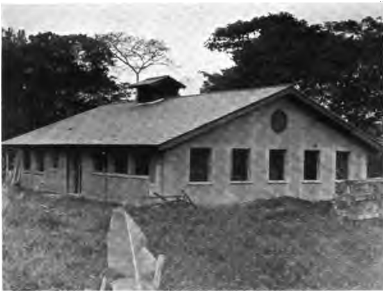
Light Plant and Laundry.
