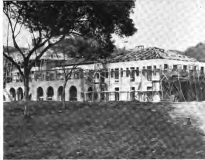
Dormitory under construction.
