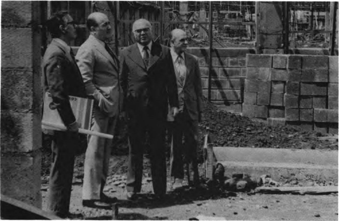
Dr. Alejandro Orfila, Secretary General of the OAS, visits the construction site of IICA headquarters building, accompanied by high-ranking IICA staff members.
