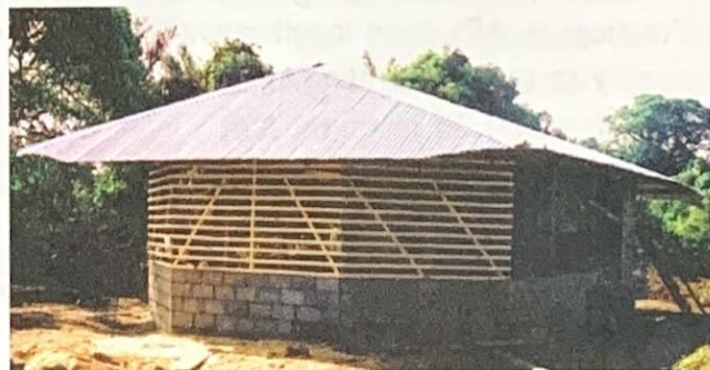
Construction of a Gangasa (Village Kitchen)
