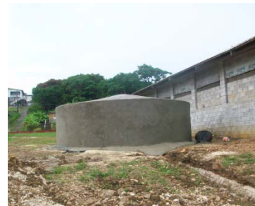
Ferro-cement tank constructed at Barnwell Farms, Rock hall, St. Thomas
