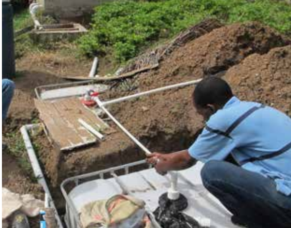
Establishing a biodigester a demonstration plot.
