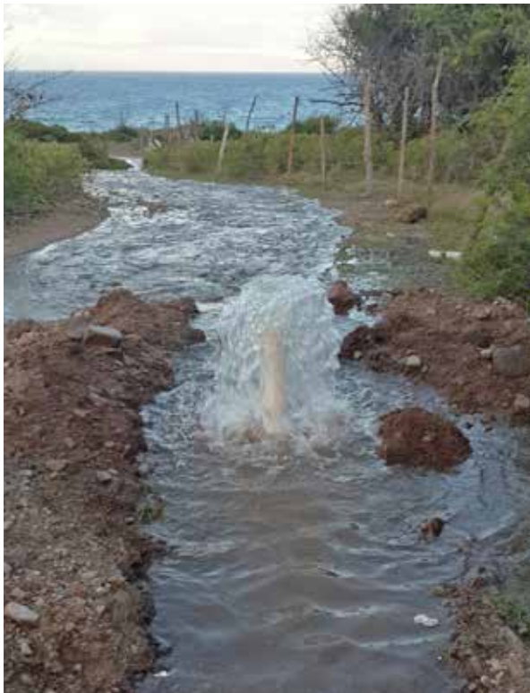
Flushing of pipe line to remove any debris before releasing water to farmers.
