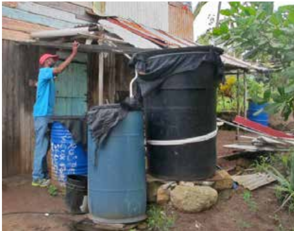
Farmer setting up rainwater harvesting system to store water on farm.
